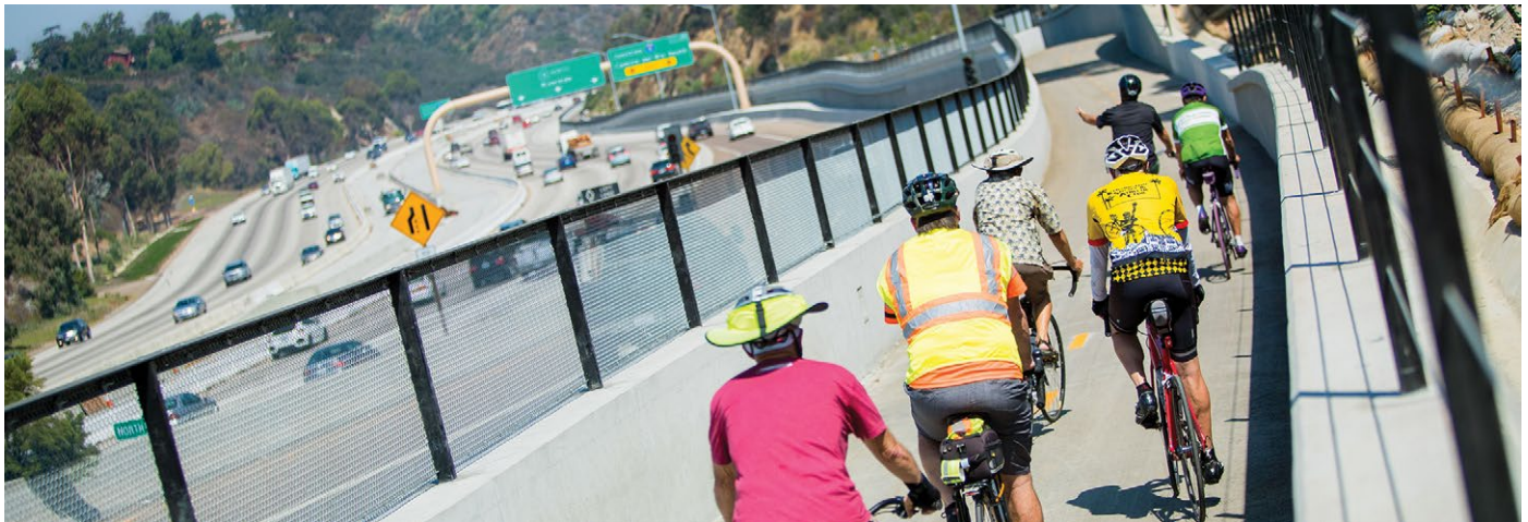
The State Route 15 Commuter Bikeway in San Diego opened to the public last August, a one-mile section connecting Mid-City communities and separated from busy SR 15. Caltrans was one of the partners in the joint project. Preliminary engineering has begun on a connecting segment.
