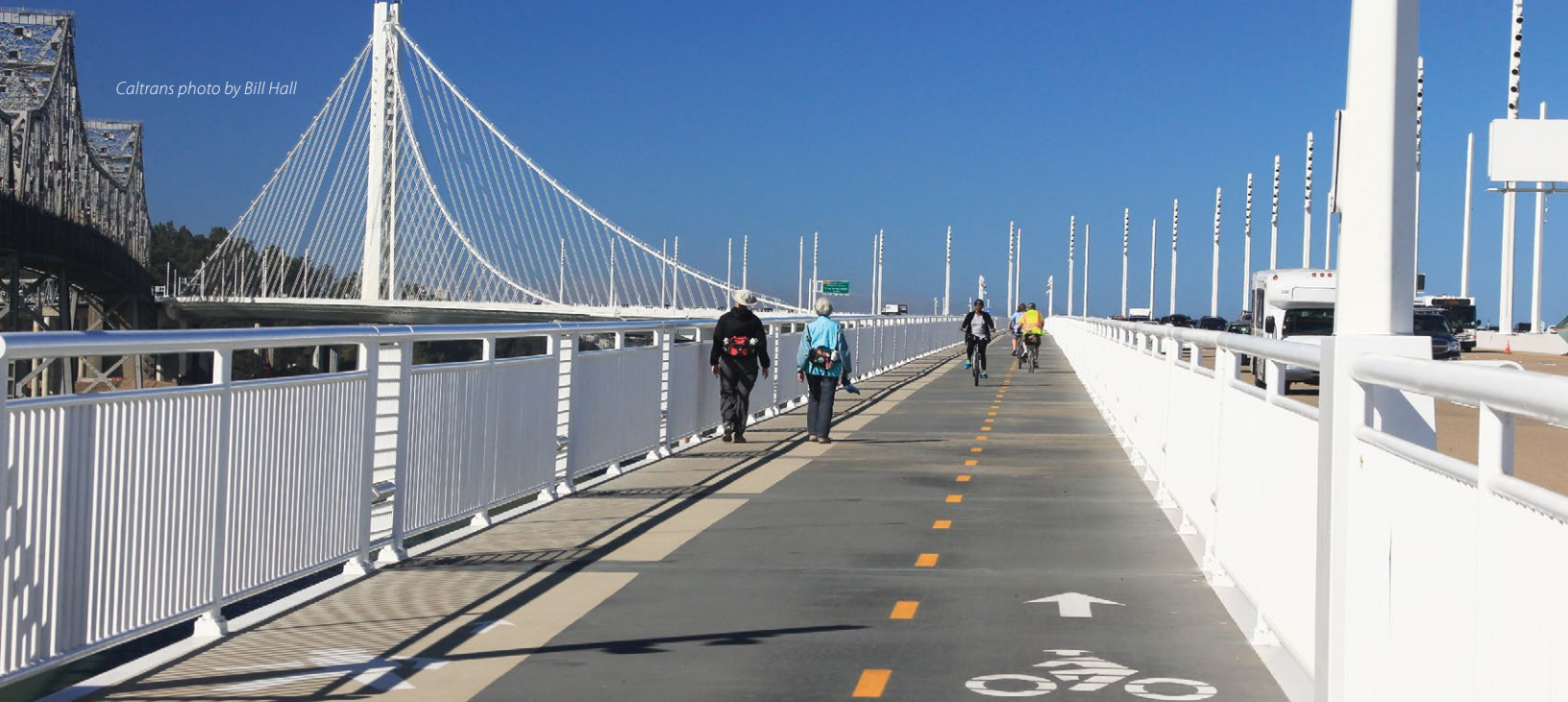
A new path for bicyclists and pedestrians across the east span of the Bay Bridge debuted in 2016 as part of the Bay Bridge Trail. The 15.5-foot-wide, striped path is among the projects that Caltrans has built and promoted as part of its "Toward an Active California" bicycle and pedestrian plan.
