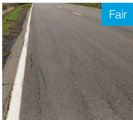
Following the new MAP-21 federal guidelines, pavement condition is rated using specific technical criteria to measure roughness, cracking, rutting and faulting.
